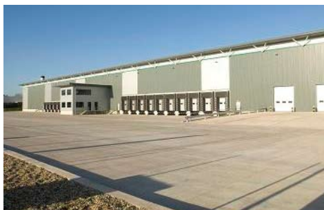
ProLogis Park Midpoint Building Three - the location for the new Biffa Super MRF.
