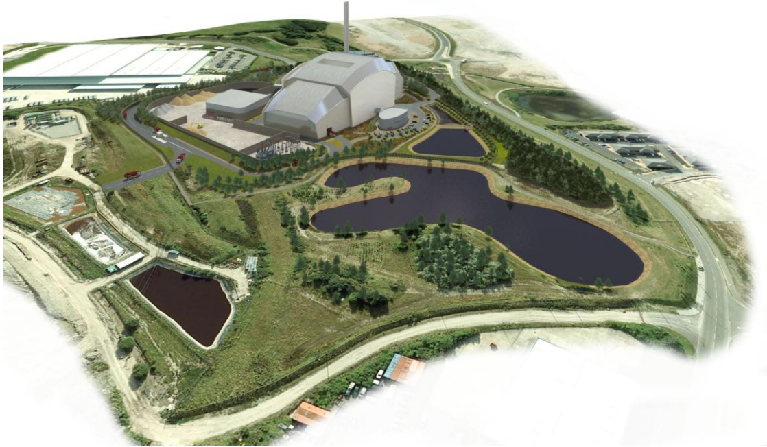
Figure 3-5 View of building looking north-west
